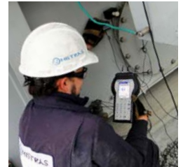
Substation Reliability Inspection
