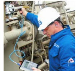
Valve Leak Detection
