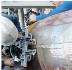
Weld Integrity Inspection
