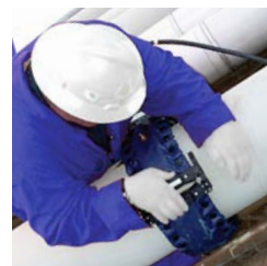
Pipeline Corrosion Inspection
